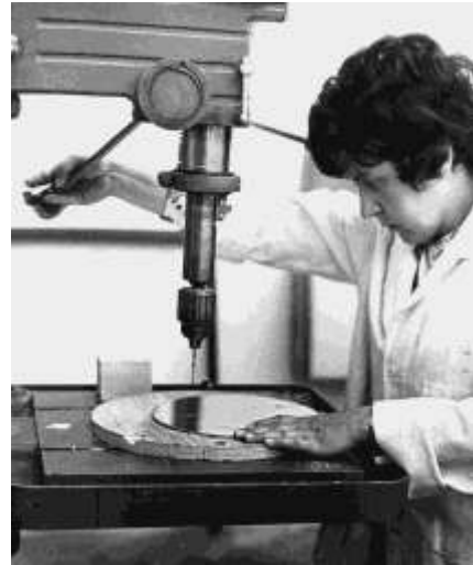
Rose drills the node of a brass gong
